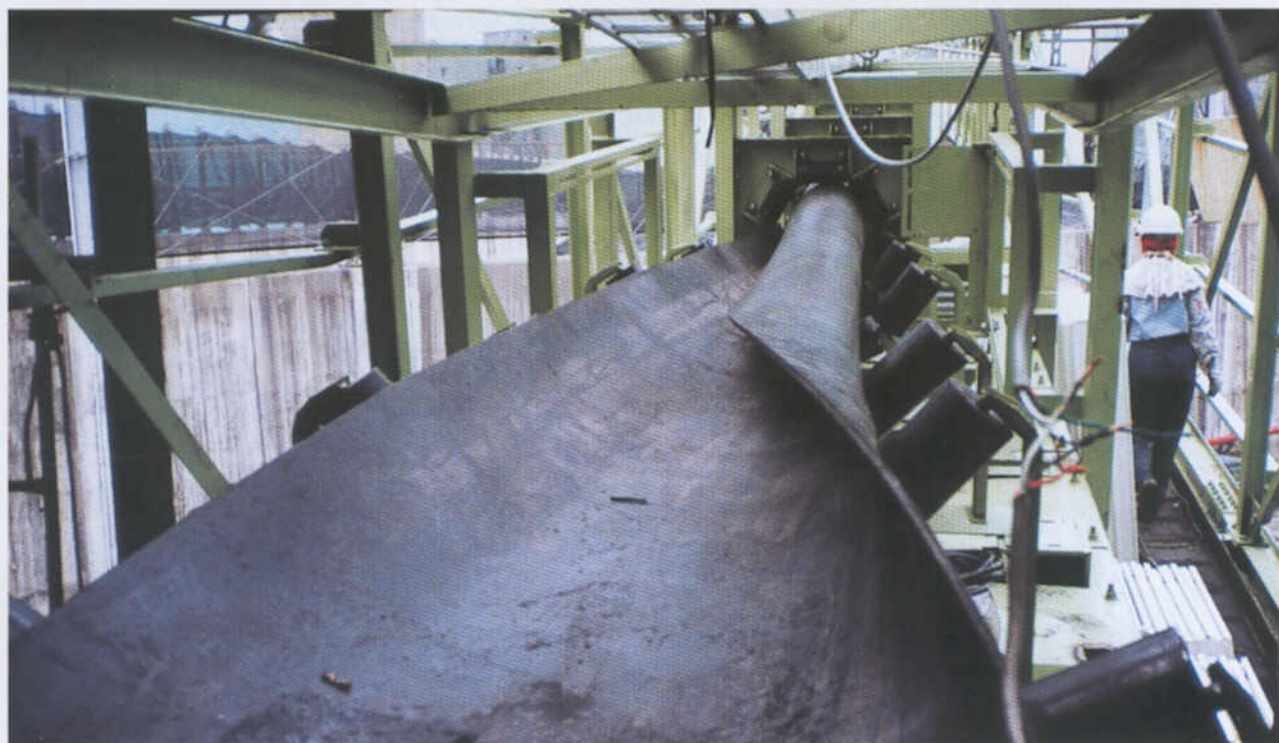
換帶作業 Removal Procedure
